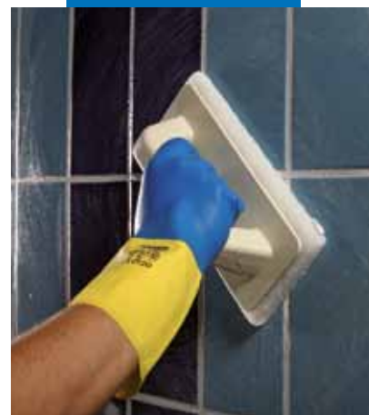
Kerapoxy CQ is emulsified with water, using a Scotch-Brite® pad
