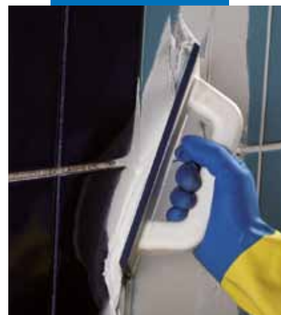
Spreading Kerapoxy CQ on a wall using a MAPEI float
