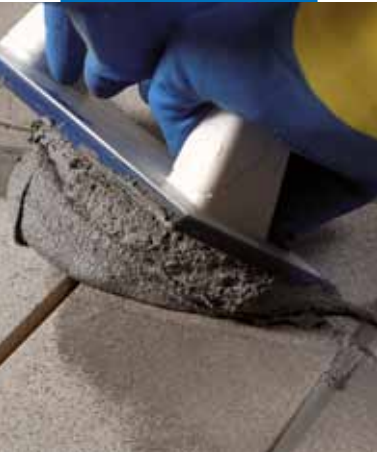
Spreading Kerapoxy CQ using a MAPEI float
