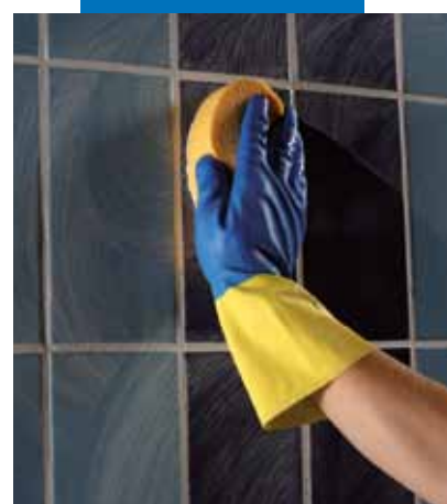
Cleaning and finishing with a hard cellulose sponge
