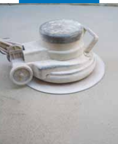
Smoothing the surface with a steel disk
