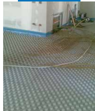
Preparation of the heating/cooling system
