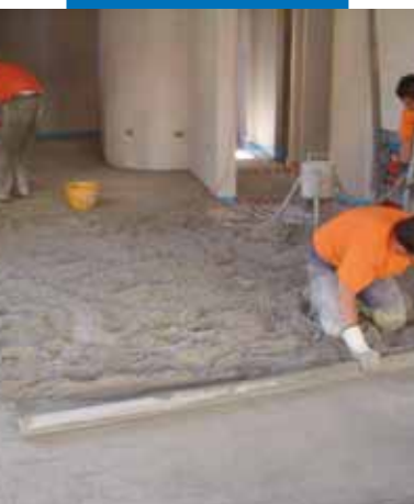
Spreading the mix with Mapescreed 704 admix
