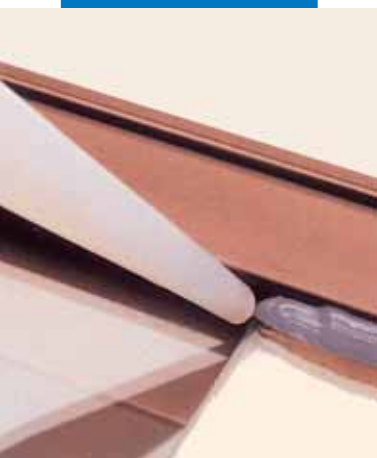
Sealing aluminium window frame with Mapesil AC
