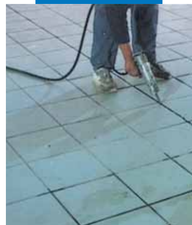
Sealing ceramic tile floor with Mapesil AC
