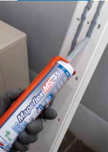
Bonding plastic profiles on a surface outside
