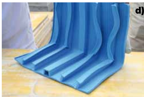
Steps to form a 90° weld in Idrostop PVC BE: a) cut the bulb and fixing lugs in the PVC BE at 45°; b) heat the two rims to be welded with the Leister; c) press the two rims together and continue heating with the Leister; d) 90° weld in the waterstop
