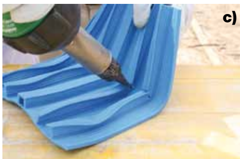
Steps to form a 90° weld in Idrostop PVC BE: a) cut the bulb and fixing lugs in the PVC BE at 45°; b) heat the two rims to be welded with the Leister; c) press the two rims together and continue heating with the Leister; d) 90° weld in the waterstop
