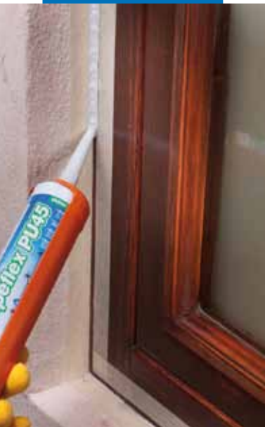
Flexible sealing of joints
