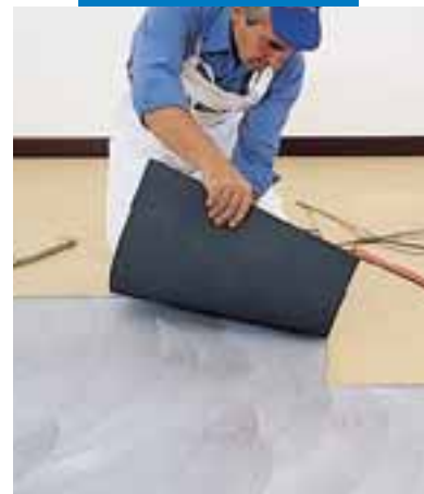
Homogeneous PVC installation
