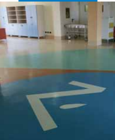
Example of PVC laid in a long-stay ward - San Martino Rest Home - Italy
