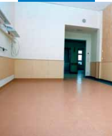
Example of application of PVC sheets - San Joseph Hospital - Germany
